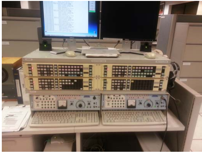
Here is what we all hear "NOAA ALL HAZARD RADIO" this console is mostly automated but can be put into a override mode if needed
